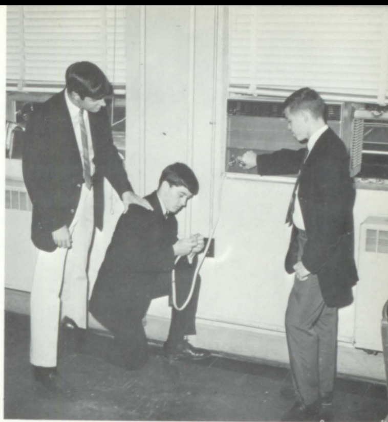
Ricky Polk, Keith Henderson, Bobby Adams check installation of air conditioner bought by council for the library.
