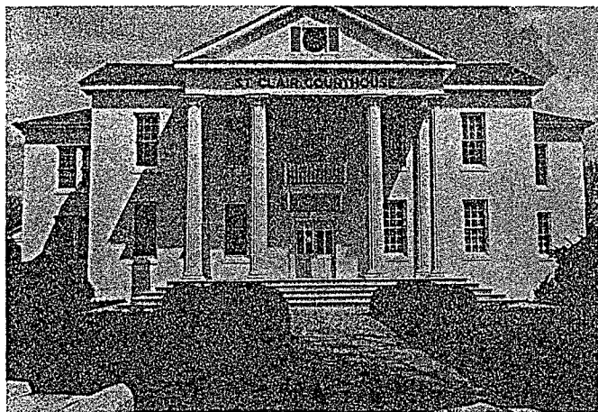
St. Clair County Courthouse
