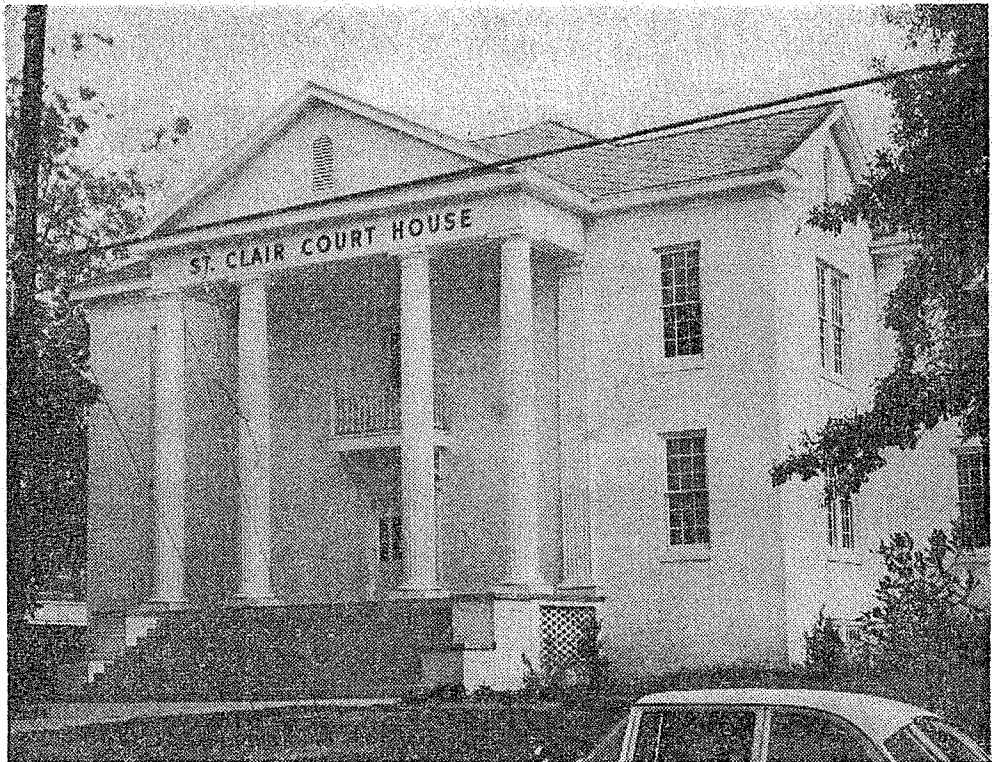
COURTHOUSE BUILT AT ASHVILLE IN 1847, REMODELED LAST YEAR ... Records in basement date back to 1819
