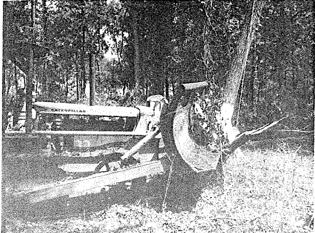
K. G. cutting blade for clearing land with bull-dozers, on the Hoyt Coupland farm, Odenville, Ala. Equipment owned and operated by Cecil Farmer, Odenville.
