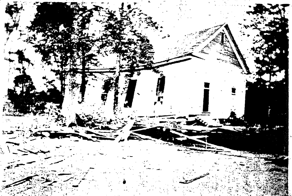
WINDS TOOK TOLE ON OLD BAPTIST CHURCH
