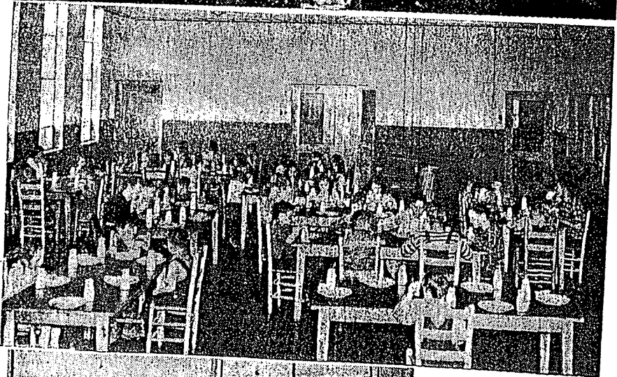
FROM The old to the new . . . views show the new and the old Eden school building. Last week
