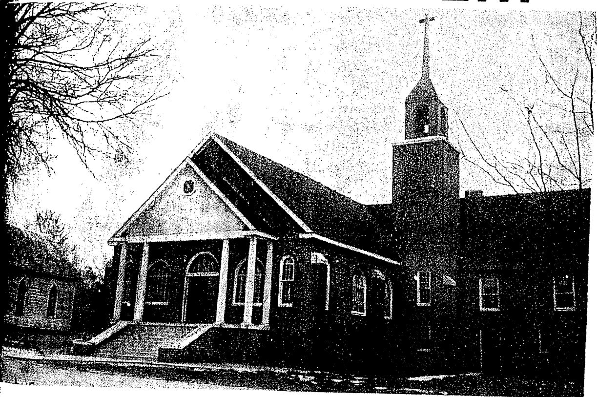
The old and the new. . Pictured is the Eden United Methodist Church, shortly after it was completed some years ago; and if you will focus your attention to the top left of the picture, you will see the old church which it replaced - which is now the Church Parsonage. Pell City Rexall has become streamlined and updated over the years, too. But...
