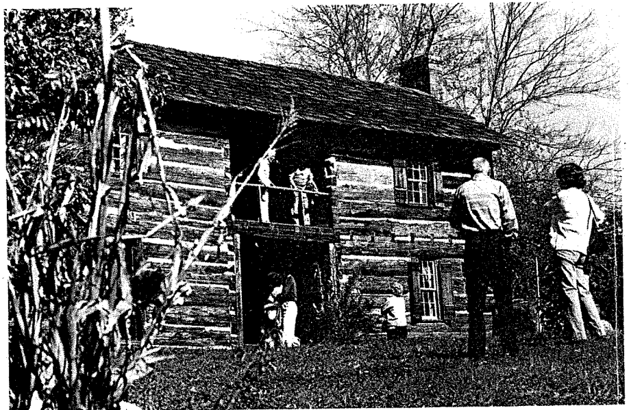
A breezeway separates the first-floor rooms, and a porch does the same upstairs, making the Looney House a double dogtrot, a rare piece of architecture in Alabama.
