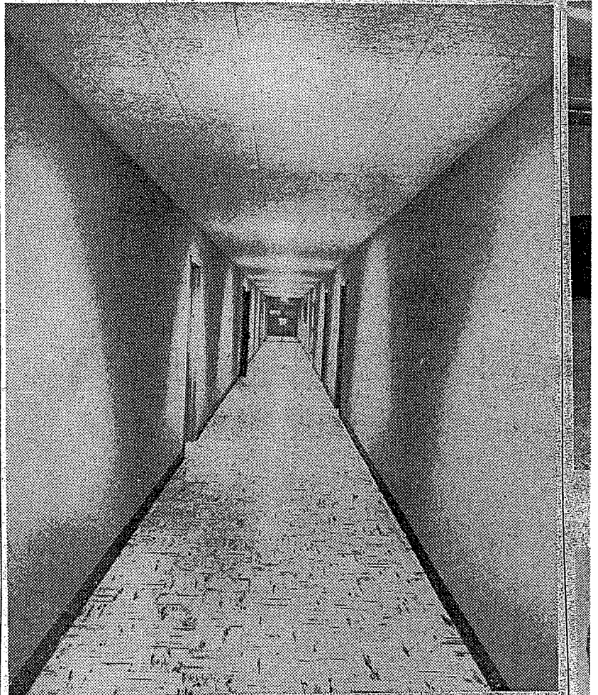
1ST FLOOR CORRIDOR
