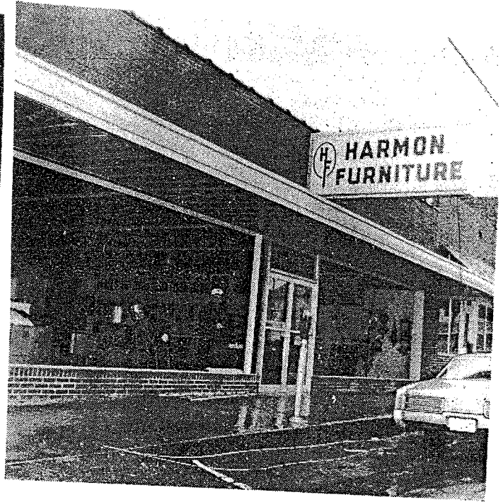
St. Clair Observer Pell City Jan. 16, 1975 Furniture Store Windows Knocked Out
