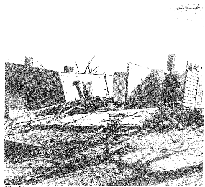
St. Clair Observer Pell City Jan. 16, 1975 Bob Rowe Home Destroyed On 1st Ave. South
