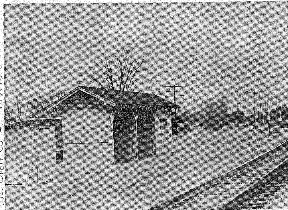
RAILWAY STATION —This tiny railroad station will also fall victim of the new lake soon to form on the present site of Riverside. The railway here will be raised several feet.
