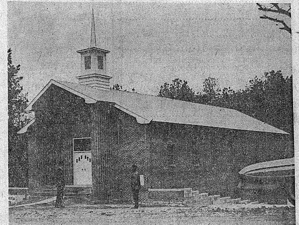
NEW $55,000 RIVERSIDE BAPTIST CHURCH ... Norman T. Cooper, left, and Mayor Coleman. Canal will be across street
