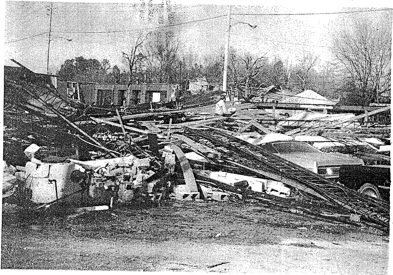
Rubble From Jan. 10 Tornado
