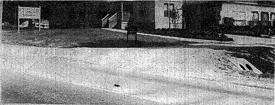
New Metro Bank construction on schedule.
