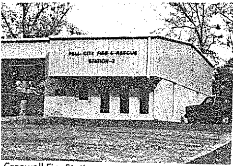
Cropwell Fire Station opened February, 1981. It is manned by two and houses the city's rescue truck, pumper and added fire protection to the southern part of our
