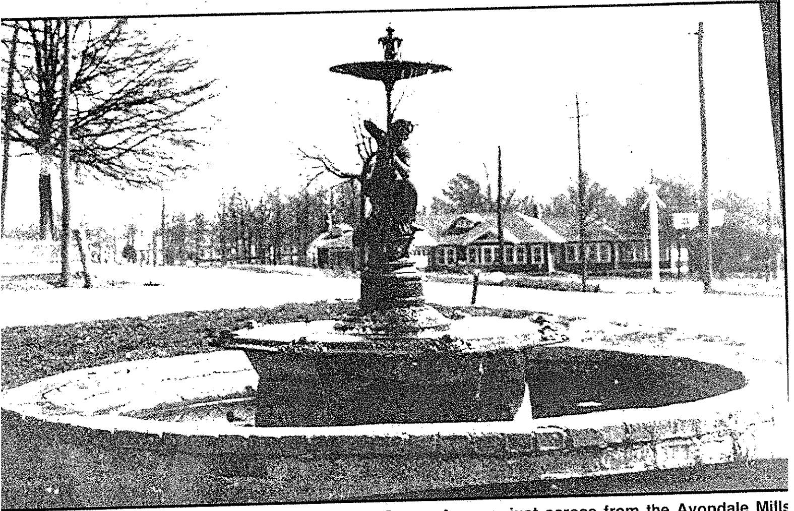
This fountain stood in the small triangle park on Comer Avenue, just across from the Avondale Mills entrance. In the background is the Avondale Clubhouse. The picture dates from around 1910. One of the goals of the Pell City Centennial Commission is to restore this fountain and the surrounding park. Avondale Mills and Gold Kist have committed their support but more is needed. The fountain was a gathering place in the summer and the commission hopes it will become a focal point for the Centennial Celebration.
