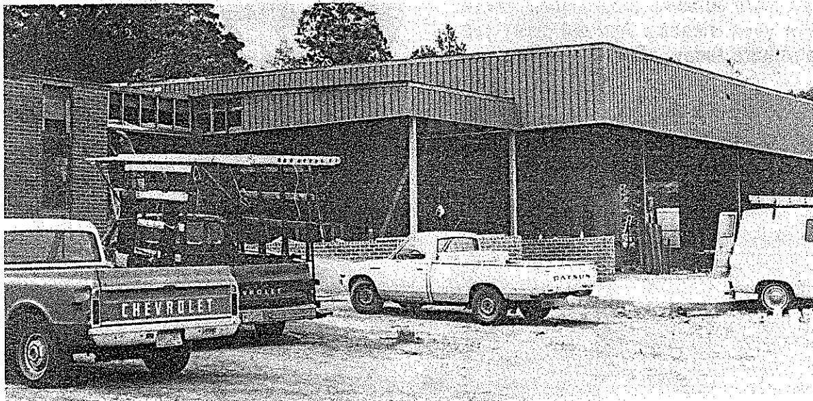
Alabama Power constructs warehouse
