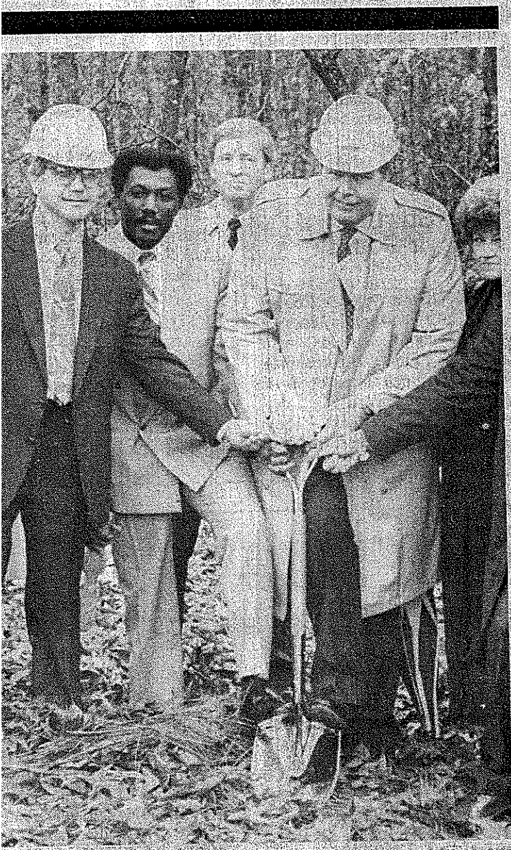
K mart ground breaking
