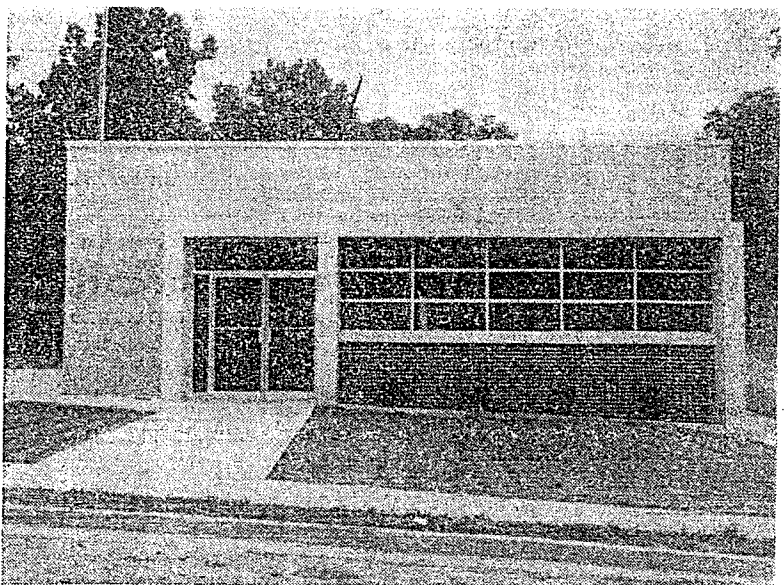
PELL CITY'S MODERN NEW POSTOFFICE
