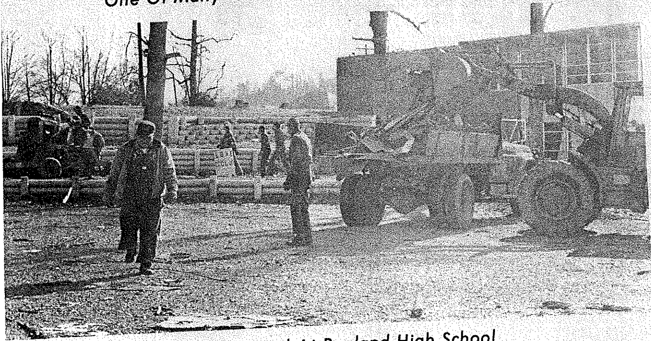
One Of Many Structures Roof-Less In Ragland
