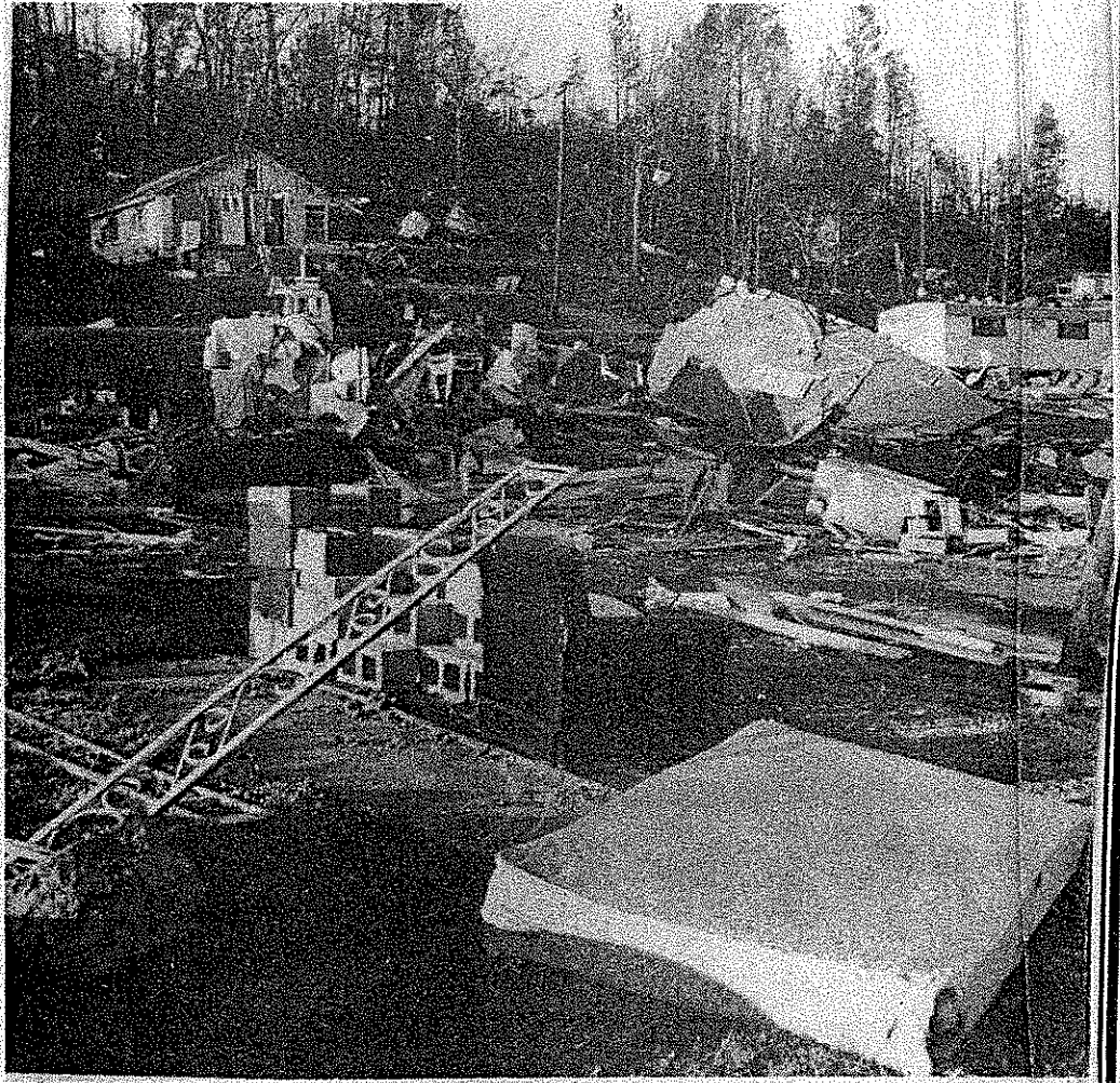
Remains of Mobile Homes At Smith Trailer Park
