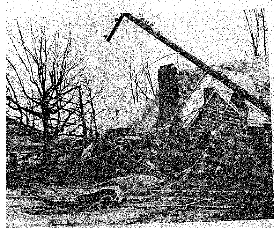
Cogswell Avenue Destruction
