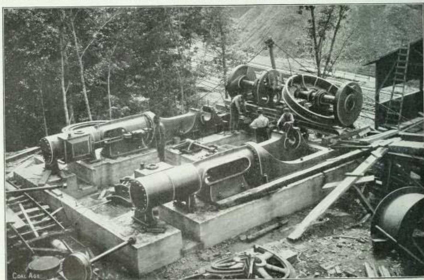
FIG. 2. THE 28x48-IN. FIRST-MOTION HARDIE-TYNES HOIST BEING ERECTED
