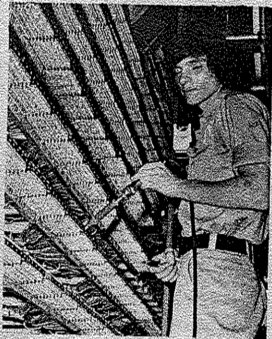
Eddy Stone Frame Maintenance
